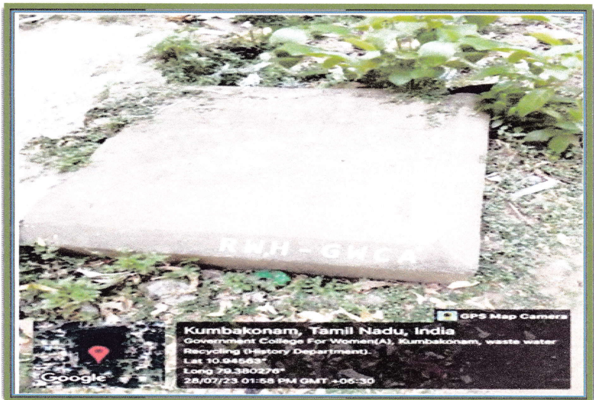
Rain water Harvesting
